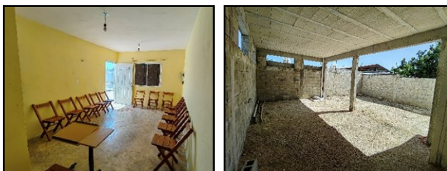
A view of the inside of the house and the large covered patio
